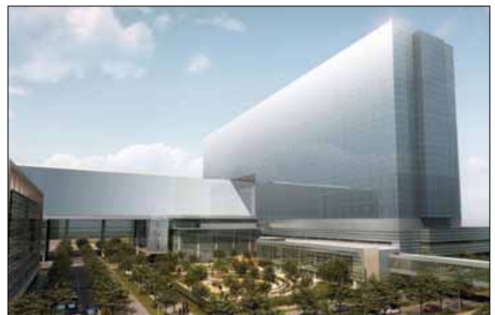
PG LifeLink Isolated Power Installation: Parkland Hospital, Dallas, Texas
